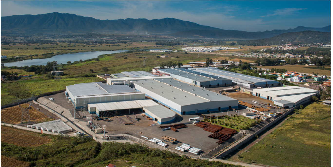
Manufacturing Plant in Guadalajara, Jalisco
